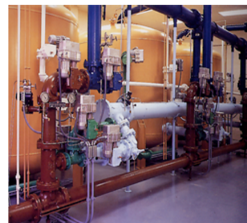
2 MGD iron and manganese filter system at work in a New Jersey municipality
