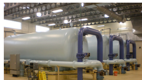
Hungerford & Terry, Inc., Clayton, NJ – pretreatment units shown above consist of three GreensandPlus™ pressure filters. Anthracite and GreensandPlus media are used to remove iron and manganese in order to protect the RO membranes.
