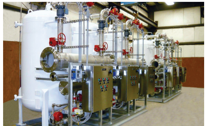
High efficiency upflow regenerated Packed Bed nitrate removal systems minimize waste and regenerant consumption
